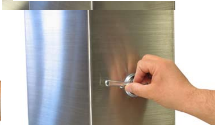
TIGHTEN THE SECURE WINGNUT TO SECURE DAMPER IN POSITION
