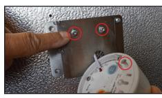
Align mounting holes on unit with mounting screw heads on bracket.
