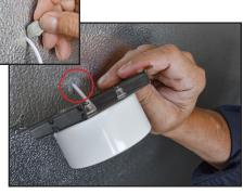
Once pulled through seal drilled hole on both sides with Permagum, to prevent air conflict.
