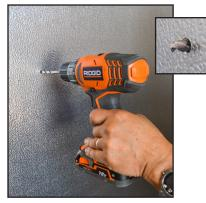
Using 5/16 bit, drill hole through panel completely through to other side.
