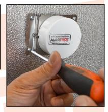
Using self tapping screws provided mount bracket to wall.
